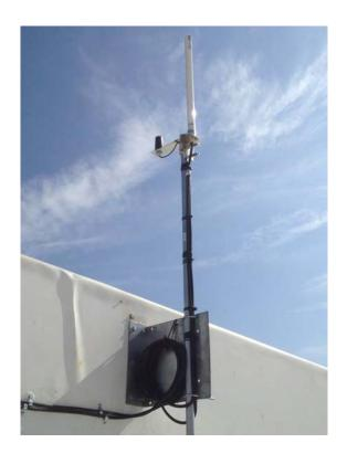
If there is more than one (1) Wireless Node in the system, you will need to install the high gain 900MHz BFA antenna and mounting bracket. The "L" bracket is designed to clear gutters. Mounting hardware and conduit is not supplied by the manufacturer.
